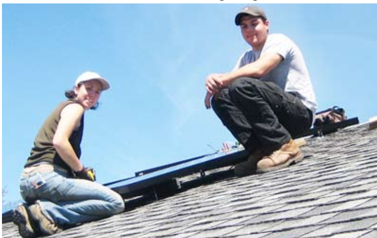
Jaye Fraser at 104 DWW with Laura of MSS laying out panels
